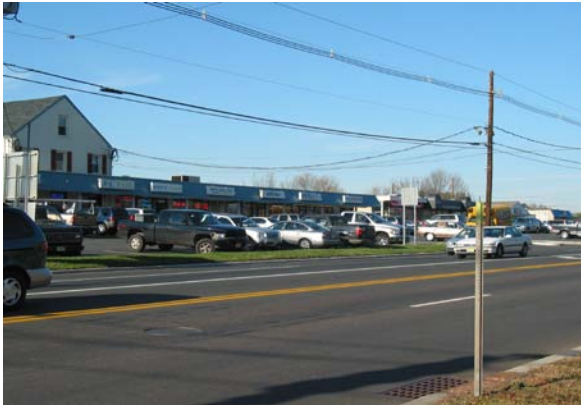
PHOTO: Typical Poor Current Condition Of Town Center Area
