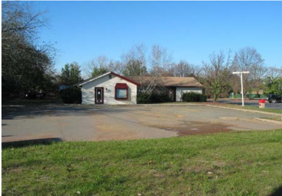
PHOTO: Existing Type of Use That Should be Replaced
