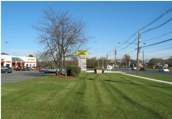
PHOTO: Inappropriate Existing Setback & Parking in Gateway A Area
