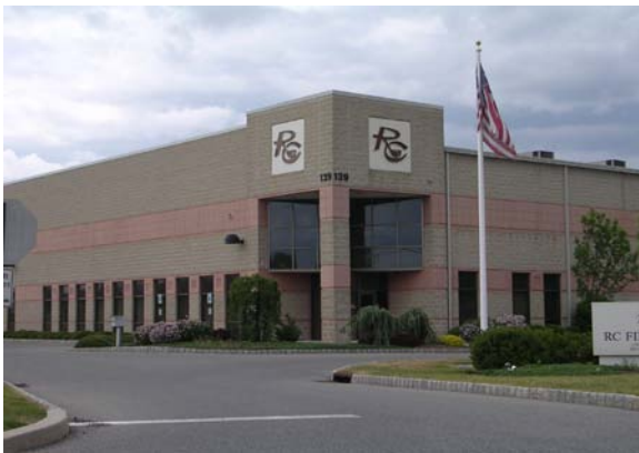
PHOTO: R&D Type Building
